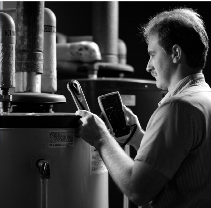
Figure 18. CO-210 w/79 Series III meter testing ambient carbon monoxide levels around hot water heaters.
