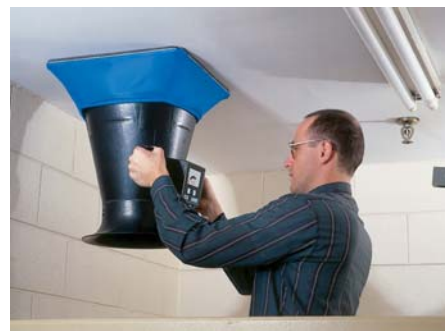
Balometer measuring a restroom exhaust
